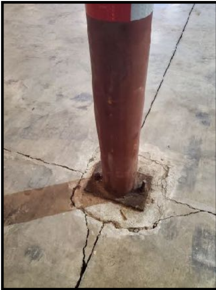
Photo 3. View of cracking around interior column
