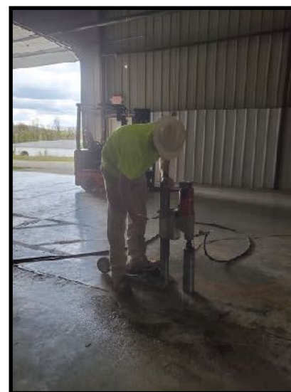
Photo 2. View of concrete coring
