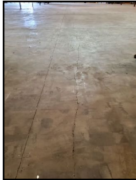
Photo 4. View of building addition area (facing west)
